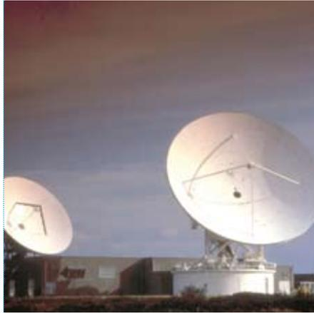
Inmarsat's Satellite Access Station (SAS) in Fuccino, Italy handles both R-BGAN and BGAN traffic. There is a second station at Burum, The Netherlands
