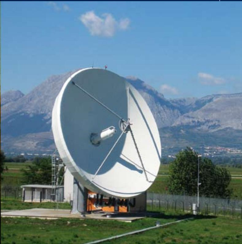
**The BGAN Satellite Access Station (SAS) is an innovative solution which provides leading-edge**, third-generation cellular services, globally via satellite. The core of the SAS is a compatible 3G cellular system which connects to the world's telephone and Internet systems. The Radio Access Network (RAN) of the SAS transmits users' voice and data, via the Inmarsat-4 satellites, to and from mobile and remote users across 85% of the world's landmass.
